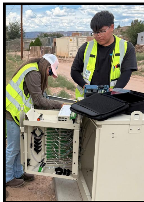
Pictured above; Keoni and Luke working at the fiber cabinet, which serves as the central distribution point connecting homes to the main fiber network.
