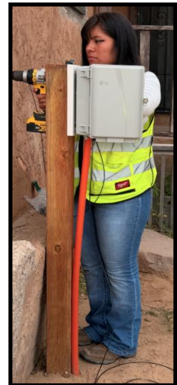
Pictured above: Kraiglyn is connecting the fiber line to the Network Interface Device (NID) and
